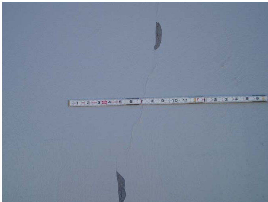
Figure 4 – Coating cracks
