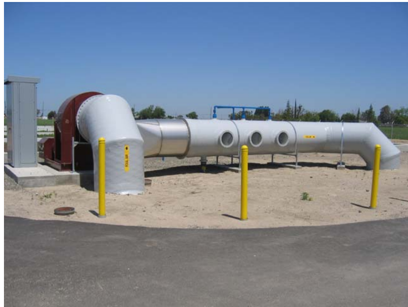
Figure 1 – Blower and In-line Humidification System
