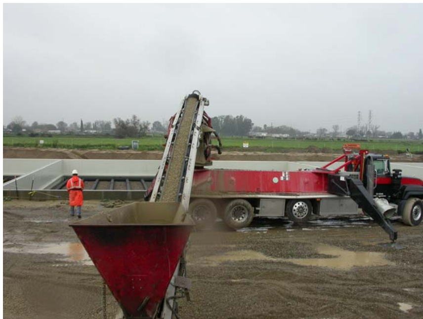
Figure 3 – Lava Rock being installed using a belt conveyor
